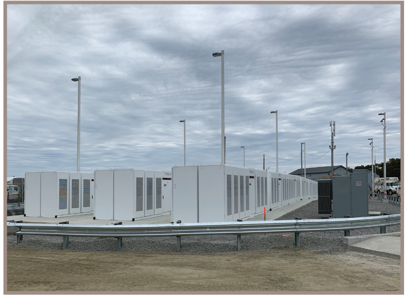
Battery Energy Storage System
